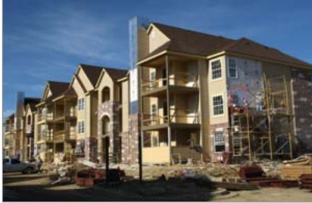
Workers brick the exterior of a phase-two apartment block of the Park at Mission Hills, a 286-unit addition to a Case and Associates complex with 308 finished units in Broken Arrow. (Rip Stell)
