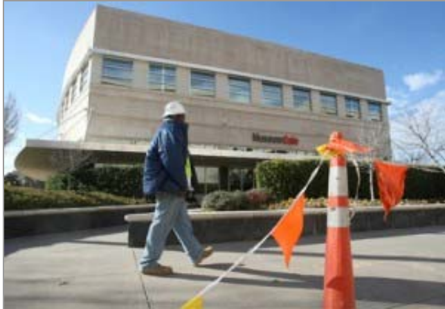
Construction in front of the Museum Cafe on Monday. (Maïke Sabolich)
