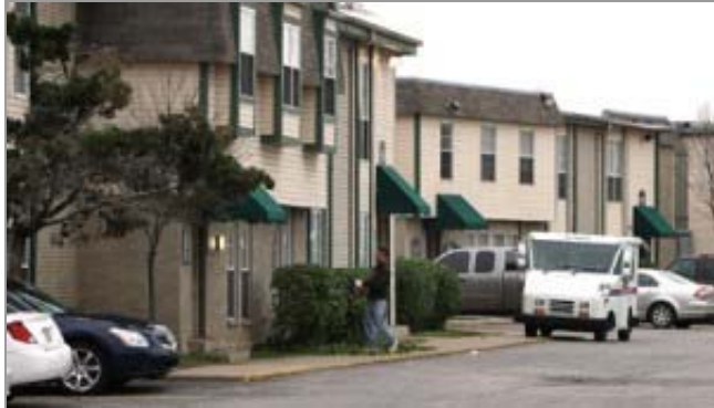
The Evergreen Park Apartments at 8314 E. 25th Pl., Tulsa. (Rip Stell)
